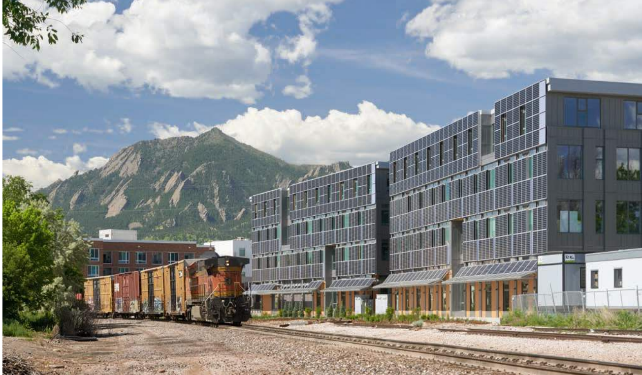
Vertical solar panels on the west side of Morgan Creek Ventures' Boulder Commons building in Boulder, CO.
